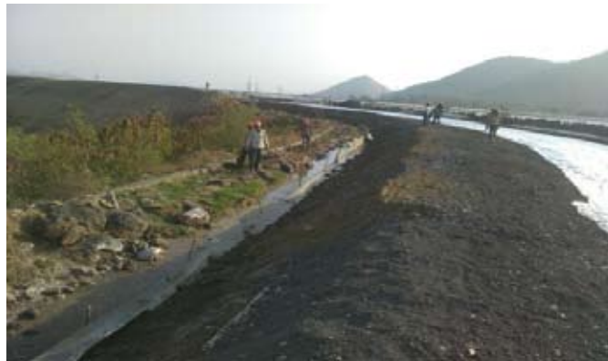
Fig. 6: Construction of embankment on geocell strengthened inner base & sheet piling
