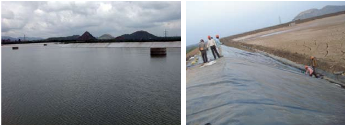
Fig. 8: HDPE liner covered with geotextile protection layer
