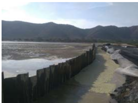
Fig. 6: Construction of embankment on geocell strengthened inner base & sheet piling
