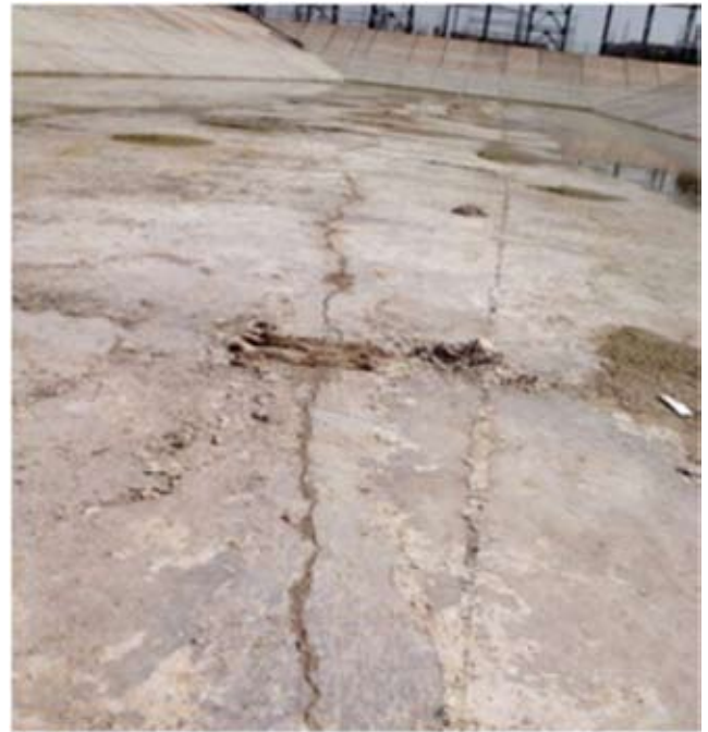
Fig. 10: Photographic view longitudinal crack at middle of reservoir base (Photograph supplied by Areva Renewable Energies India Pvt. Ltd.)
