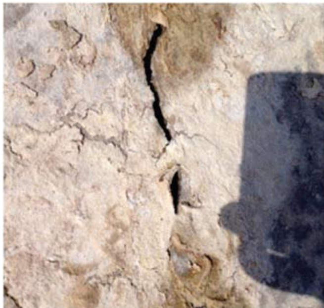
Fig. 12: Photographic view random alligator cracks at reservoir base (Photograph supplied by Areva Renewable Energies India Pvt. Ltd.)
