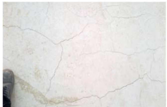
Fig. 11: Photographic view random alligator cracks at reservoir base (Photograph supplied by Areva Renewable Energies India Pvt. Ltd.)
