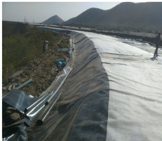
Fig. 7: HDPE lining on outside raised portion of the dyke
